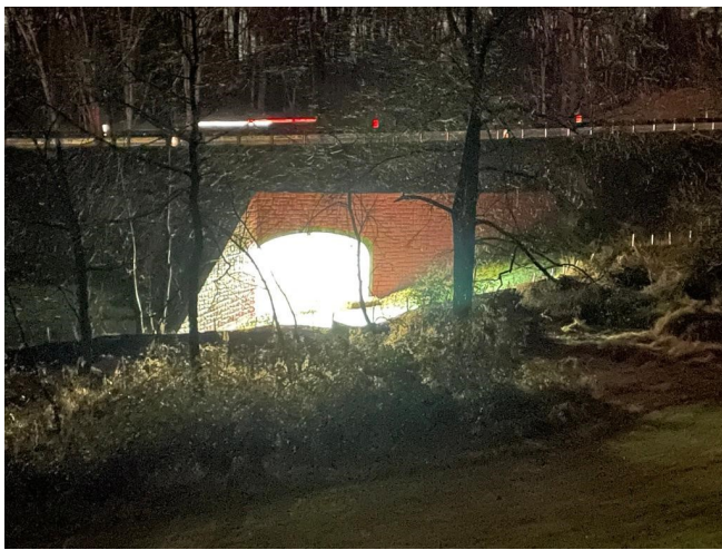
Route 7 Tunnel as part of Colvin Run Mill site
